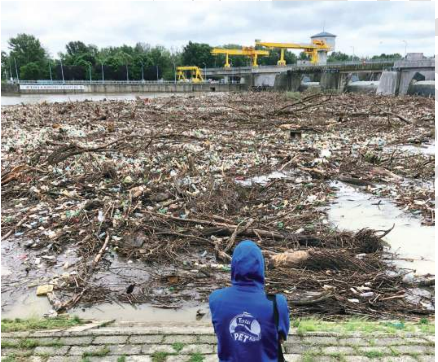
Drift wood mixed with plastic waste caught by the Kisköre hydropower dam, Hungary, spring 2019
