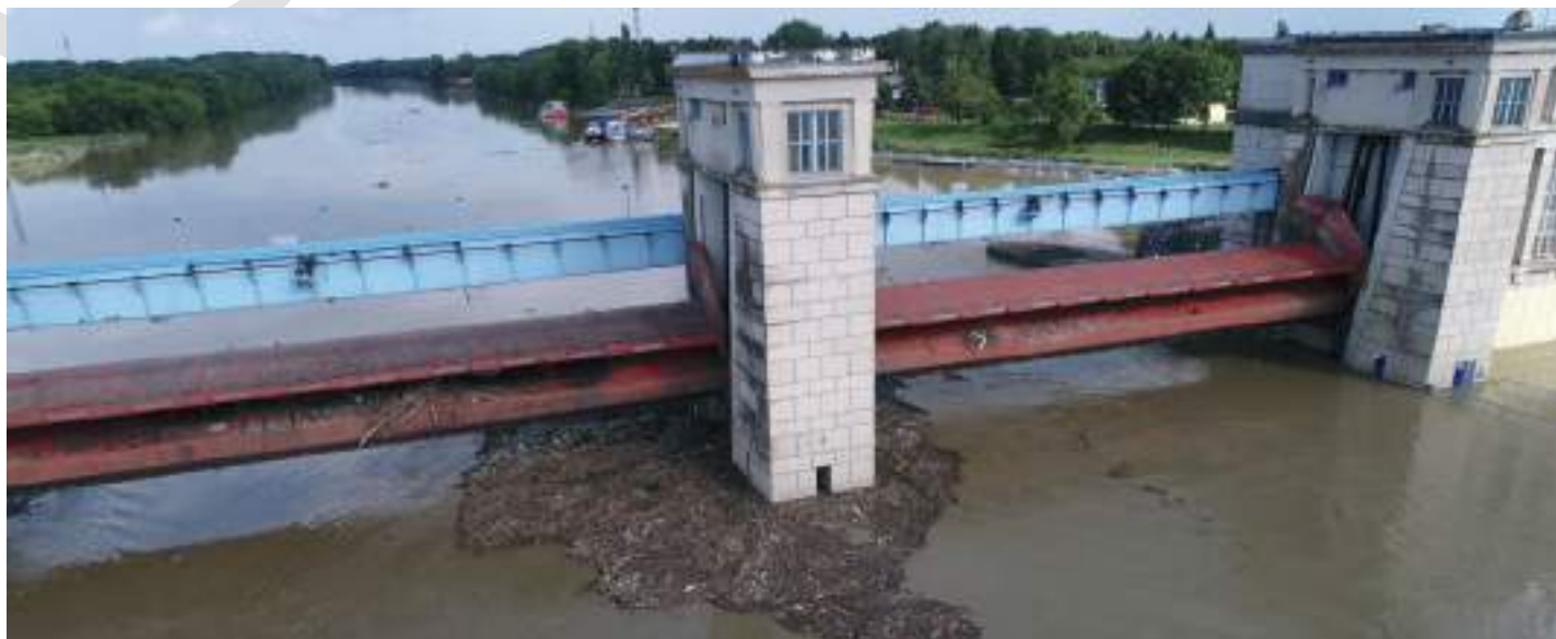
Driftwood and communal waste trapped by the Tiszalök dam, Hungary, spring 2019
