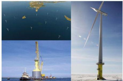
Frozen... The 2.3MW pilot turbine (right) is sited off Finland, testing the arctic weather conditions on the turbine and steel caisson foundations (left) ahead of installing the country's first commercial offshore project (top)
